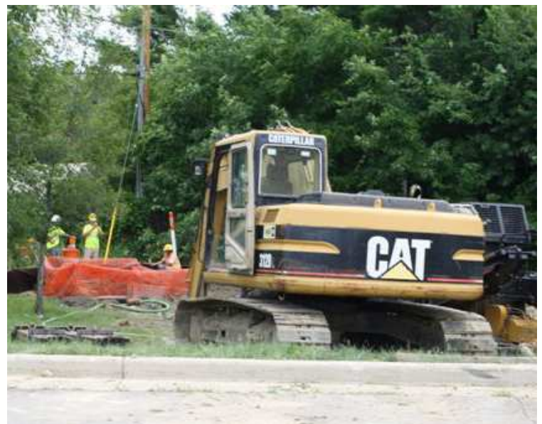
Adding the sewer pipe under Cleveland Avenue
