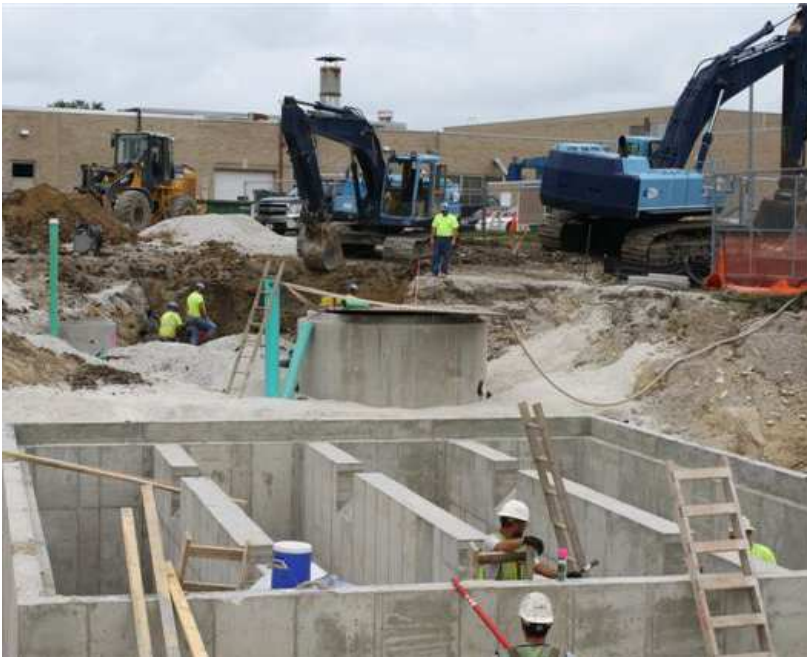
Building the sewer holding tank
