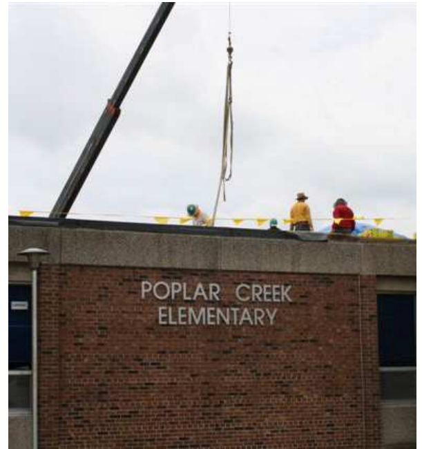
Roof Maintenance at Poplar Creek
